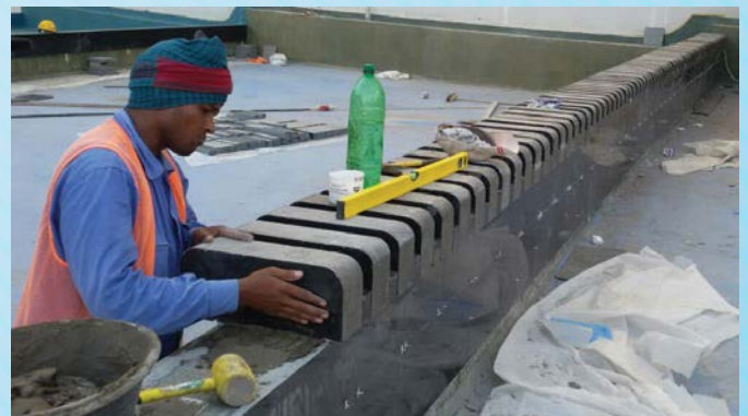
Granite coping stones were carefully fixed back in position to line and level
