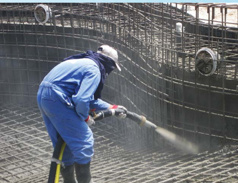
Typical dry gunite application
