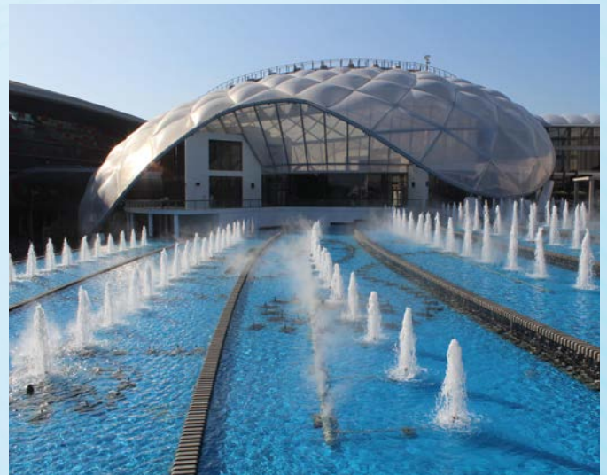
Cascade Nozzles with Fog System were introduced
